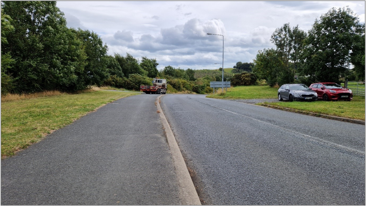
Figure 2-10 – Poor Visibility at Proposed Bus Stop
